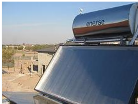
Roof-mounted close-coupled thermosiphon solar water heater.
