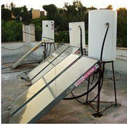
Passive (thermosiphon) solar water heaters on a rooftop in Jerusalem
