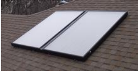
Flat-plate solar thermal collector, viewed from roof-level
