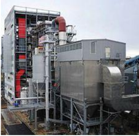
A CHP power station using wood to supply 30,000 households in France
