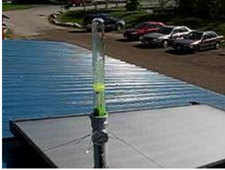
The bubble separator of a bubble-pump system
