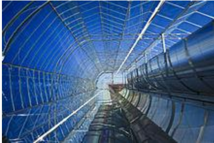
Inside an enclosed trough system
