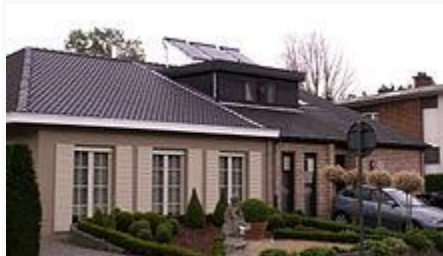
A solar water heater installed on a house in Belgium
