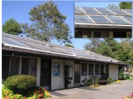
A laundromat in California with panels on the roof providing hot washing water.
