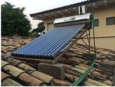
Evacuated tube solar water heater on a roof
